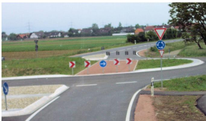
One other solution could also be a lane built in a direct line across the central island. The picture shows an example next to the factory Herrenknecht which transports their extremely large tunnel boring machines to the next harbour via this road.
