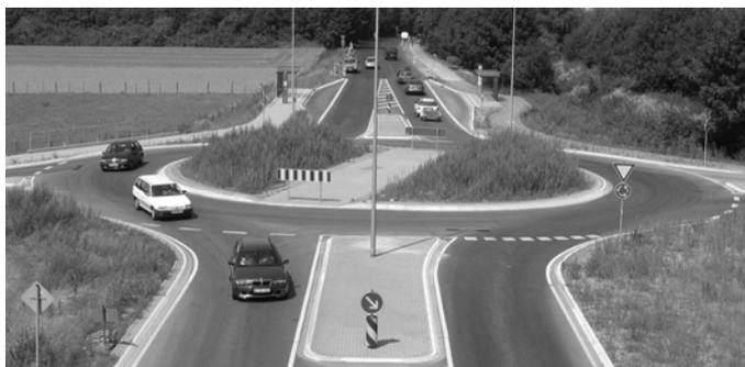
One solution which is mentioned by the picture (on the left) in the guideline from 2006 is a lane crossing the centre island from left to right. Here the big truck approaches the roundabout not on the entry lane but via the exit to leave the roundabout via the ordinary exit of his direction. The advantage is that normal traffic is approaching the roundabout looking on the green part of the island and thus keeping the drivers alert of the roundabout.
